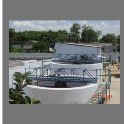
Industrial Effluent Treatment Plant
