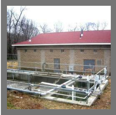
Sewage Treatment Plant
